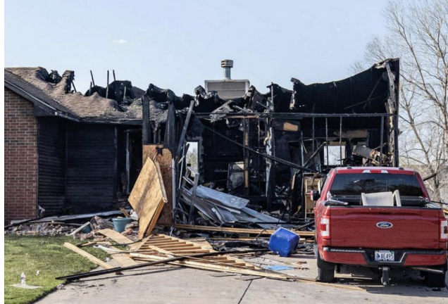
THE AFTERMATH (note the house's brick facade)
